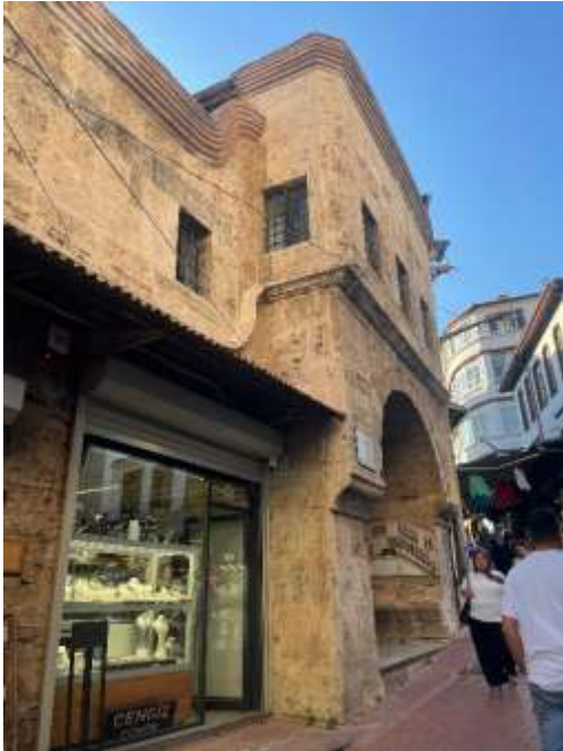
Figure 4. Entrance area of Yukarı Taşhan
